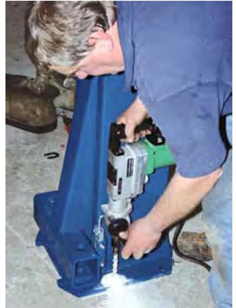
Once the columns are right where they need to be, Dennis uses a masonry drill to make the holes in the floor. The dimensions of the holes are another specification that should be verified per the lift manufacturer's instructions, as the anchors are designed for a specific diameter hole. The better the concrete, the longer it takes to drill each hole.
