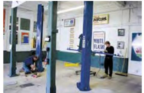
With the lift columns secured to the floor, all that remains is to assemble the unit. Most of the remaining steps are simpler to perform than the actual placing and mounting of the columns, though you'll still need power. Nearly all lifts require a 220-volt source—do not attempt to run yours on 110. We had an electrician handle our wiring, and added a lockable service box next to the lift to shut off the power feed in case of emergency or to prevent untrained users from messing with the unit.
