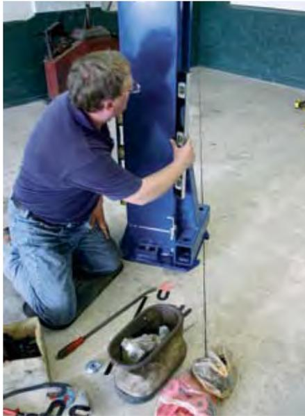
Prior to drilling any mounting holes, Dennis gets both columns in precisely the correct position. This includes dialing in the vertical attitude of each column using shims. Our Bend-Pak lift came with a shim pack, but Dennis had a variety of his own. Since each column mounts independently, the pair must be parallel so that the lift arms don't come under stress as the vehicle is lifted.
