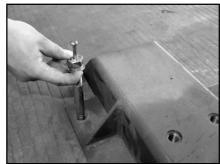
Fig. 3 A, B, C (Anchoring Base Plate)
