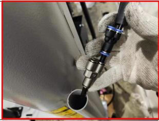
CONNECT THE BLACK AIR HOSE FROM THE ASSIST ARM TO THE T FITTING
